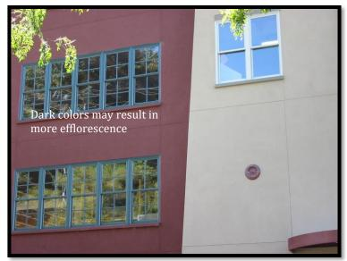
periods of damp and cool weather followed by warm sunshine can lead to efflorescence. If the color of the wall is dark, the wall heats up and can accelerate the evaporation process drawing more salts to the surface. Caution should be given to owners selecting dark colors as efflorescence might increase.
